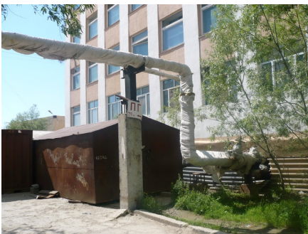
Utility lines in a permafrost zone must be above ground
