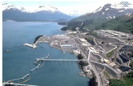
Valdez Oil Terminal
